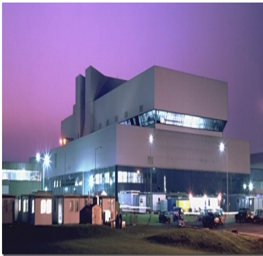
JET facility at Culham (Source: EUROfusion)
